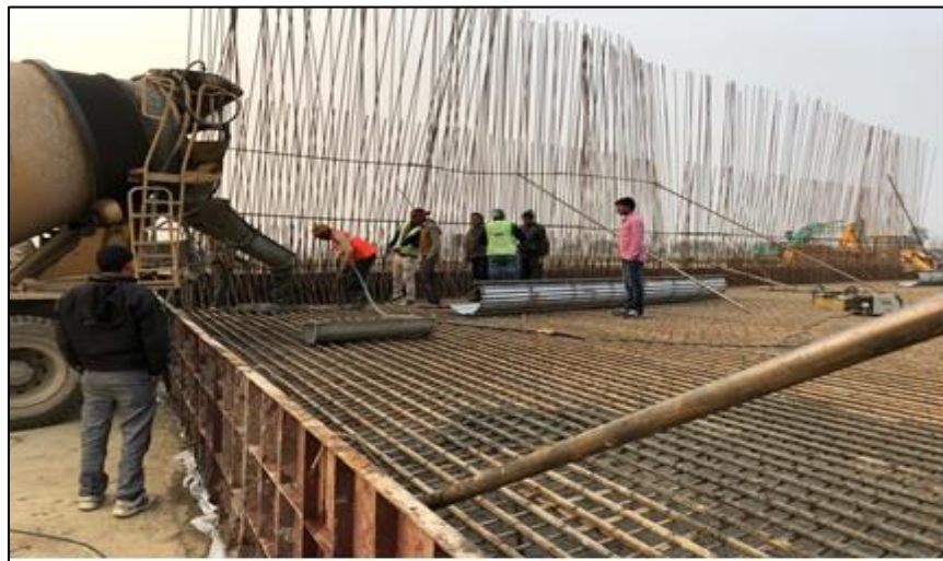
Fig. 0.3 – Construction of Purvanchal Expressway
