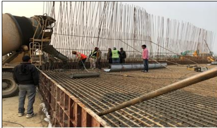
Fig. 0.3 – Construction of Purvanchal Expressway
