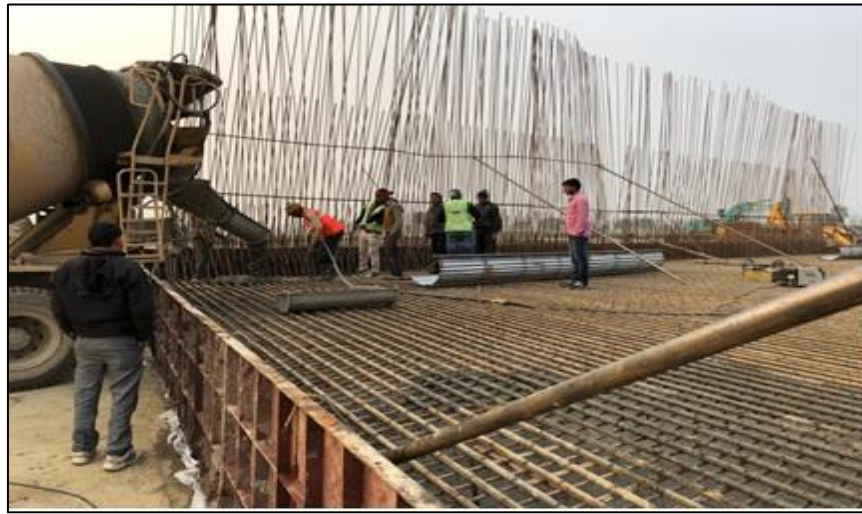
Fig. 0.3 – Construction of Purvanchal Expressway
