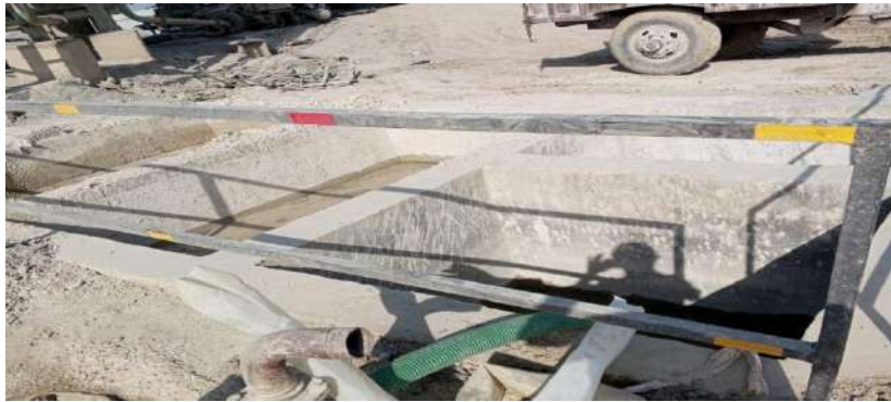
Sedimentation Tank to Contain effluent Discharge from Concrete Batching Plant
