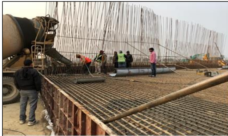
Fig. 0.3 – Construction of Purvanchal Expressway
